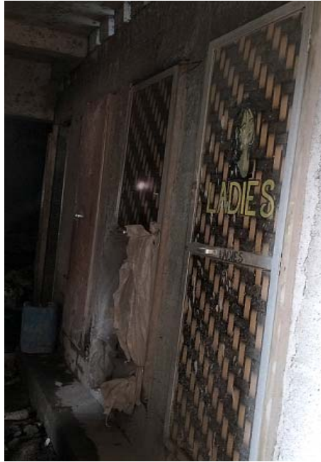
OWC INSTALLED ON SITE
